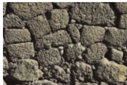
Aparelho poligonal – muralha Polygonal gear – wall
